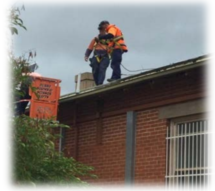
Installing solar panels
